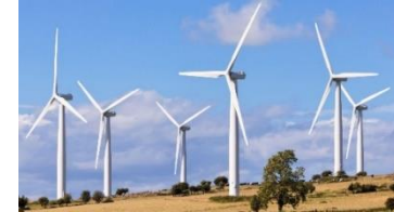
Wind Farm Control
