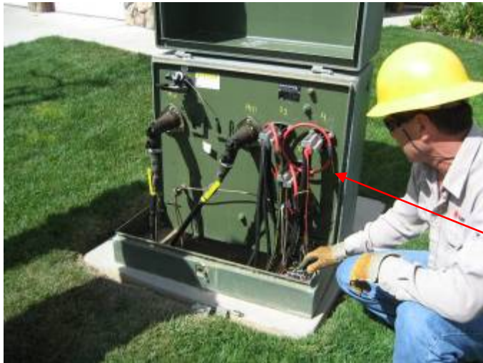
Monitoring on Distribution Transformer
