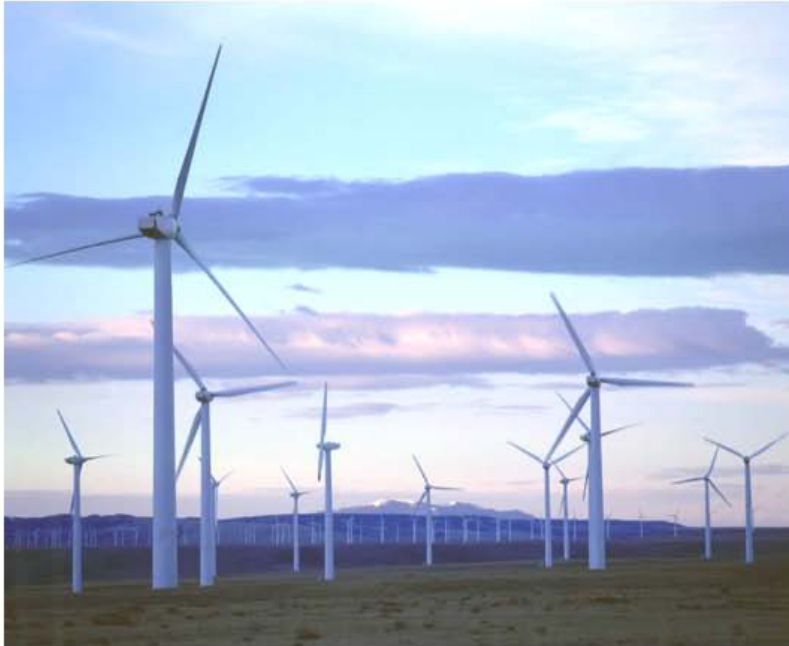
Shell's Rock River windfarm in Carbon County, Wyoming, USA Source: http://www.the-eic.com/News/Archive/2005/May/Article503.htm
